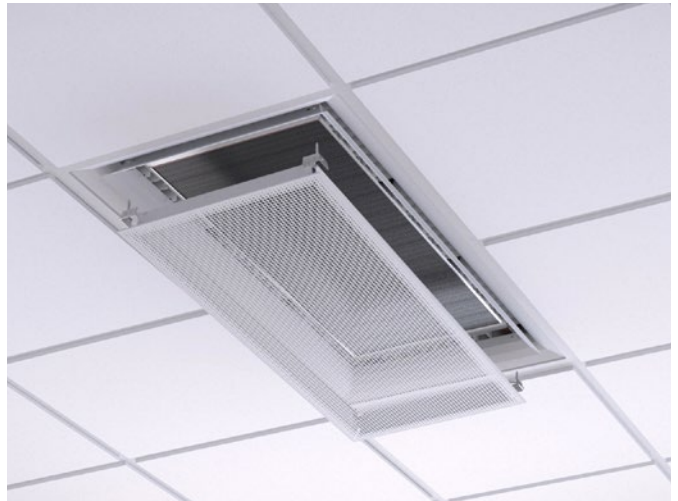
Figure 14. Removing the face plate to access the coil
