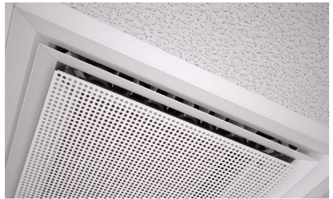
Figure 10. Standard face plate Circular holes arranged in a square pattern
