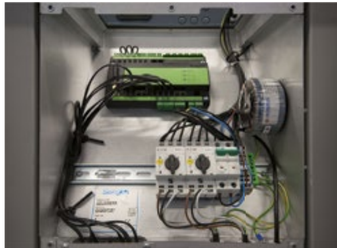
All electrical and control equipment is collected inside a special enclosure in the centred section of the air handling unit.
